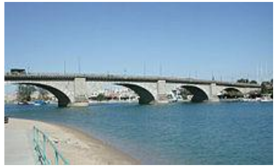
Lake Havasu City Bridge, Arizona
