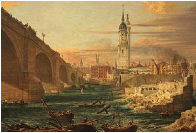
Demolition of old London Bridge
