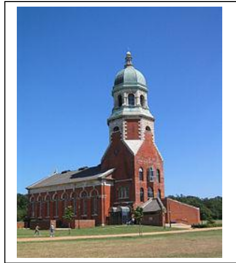
The Hospital Chapel (still surviving)
